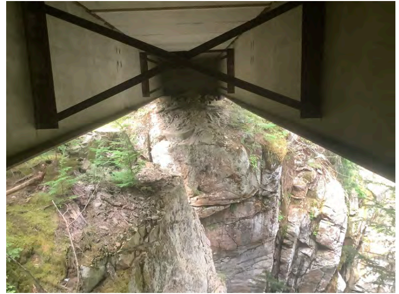
Right Bank Abutment when facing downstream
